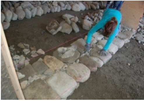
Laying the foundations
